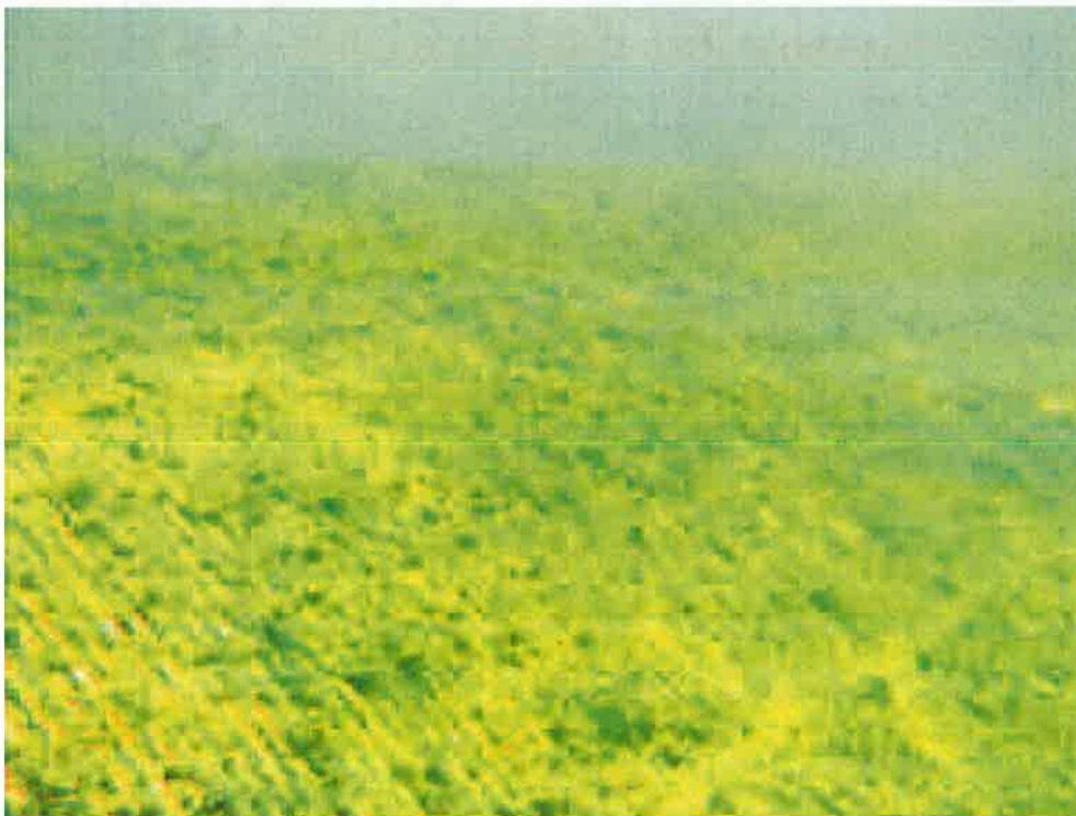
Figure 3. Algae on all upper surfaces of screen cylinders. The amount of algae observed is typical for a shallow screen on the Sacramento River and will not appreciably restrict water flow.
