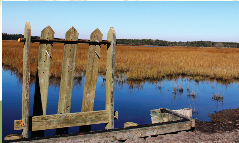
This new rice trunk water control structure on Bear Island WMA was installed by leveraging SCCB match to secure a NAWCA grant for the area.
